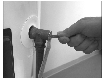
Figure 13 - T&P Relief Valve
